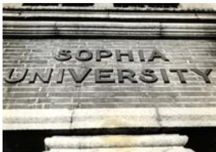
3. The entrance to Building No. 1, showing the school name in bronze letters (this feature no longer exists).
