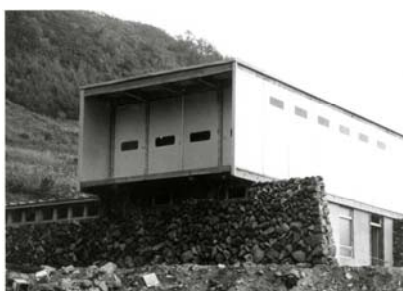
The original Hōdaigi Lodge (completed November 1963). The first story was made of stone and the second story was covered with aluminum siding.
