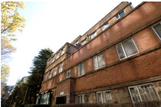
A recent picture of Building Number 1
