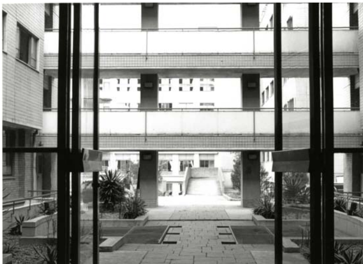
Seen from the old library building, this picture shows the outdoor connecting area, with the ventilation grates needed for the Law Building.
