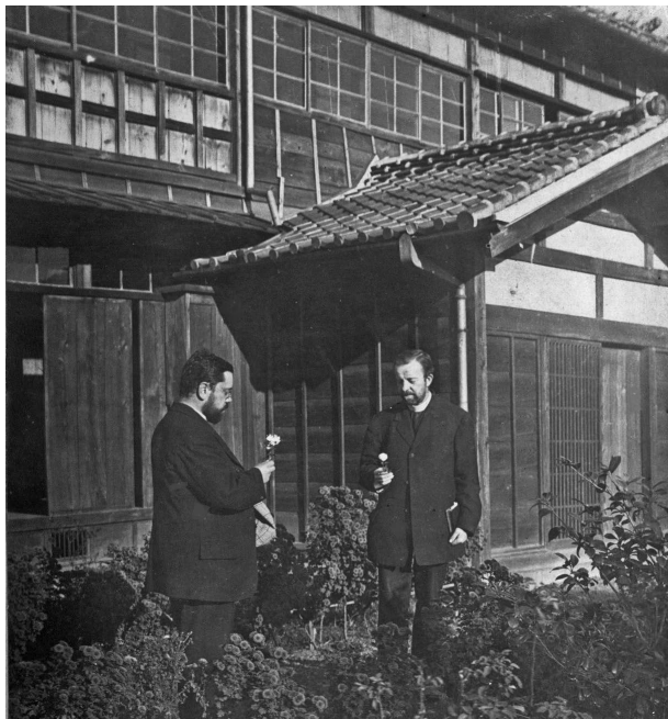
Figure 8. The Myōgadani residence used by the Jesuits from November 1908 to June 1912. In the foreground, Victor Gettelman (left) and Hermann Hoffmann. Sophia Archives.
